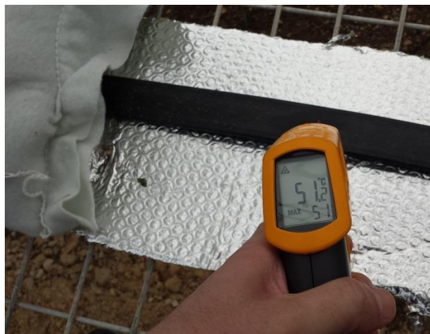
Heating Ribbon under the perlite substrate
