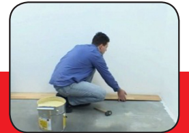
INSTALL FLOOR COVERING
